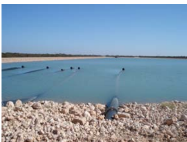
Pump Shed and 500 megalitre dam at Boundary Bend Olives
