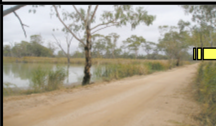
Before - 3 large pipes allowing for water flow
